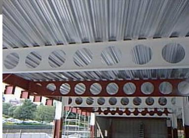
*40 to 55% of beams can be left unprotected by placing protection where it is needed.*
